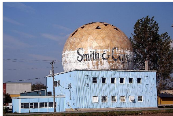
Figure 8: Radar Dome, Current Condition
